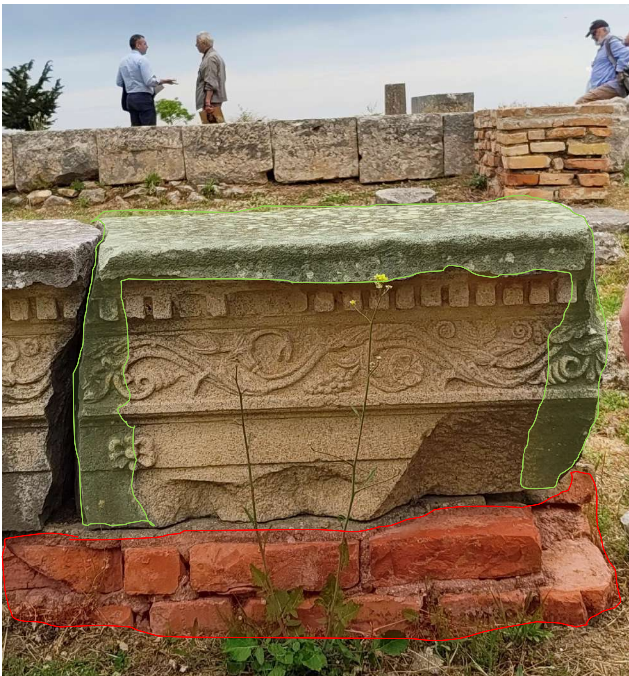
Figure 36 Decorated erratic elements scattered around Bylis theatre, poorly arranged and affected by biological patina and erosion; requires cataloguing and relocation for proper conservation.
