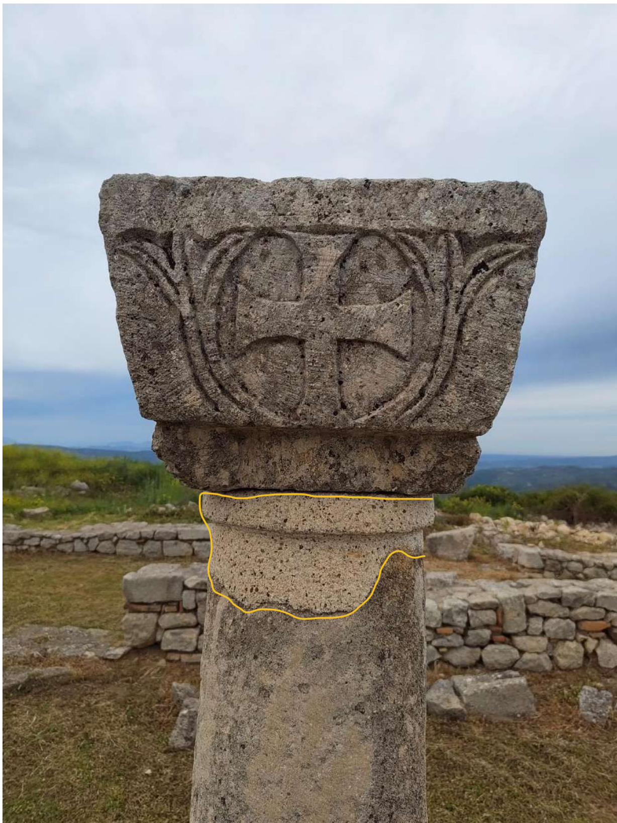
Figure 34 Reconstruction of a portion of the column using incongruous material.
