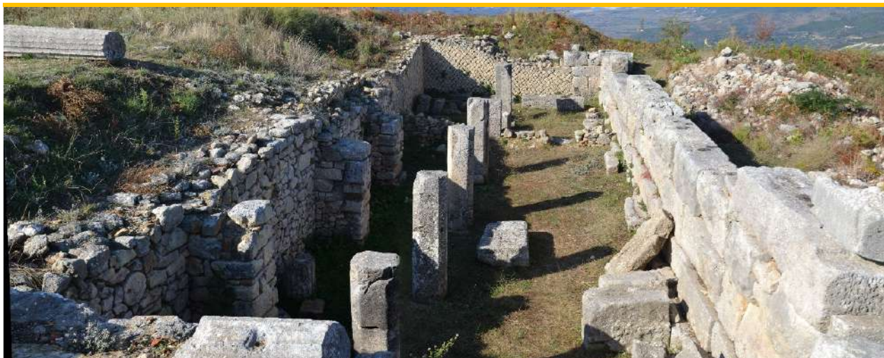
Figure 26 Arsenal after the restoration
