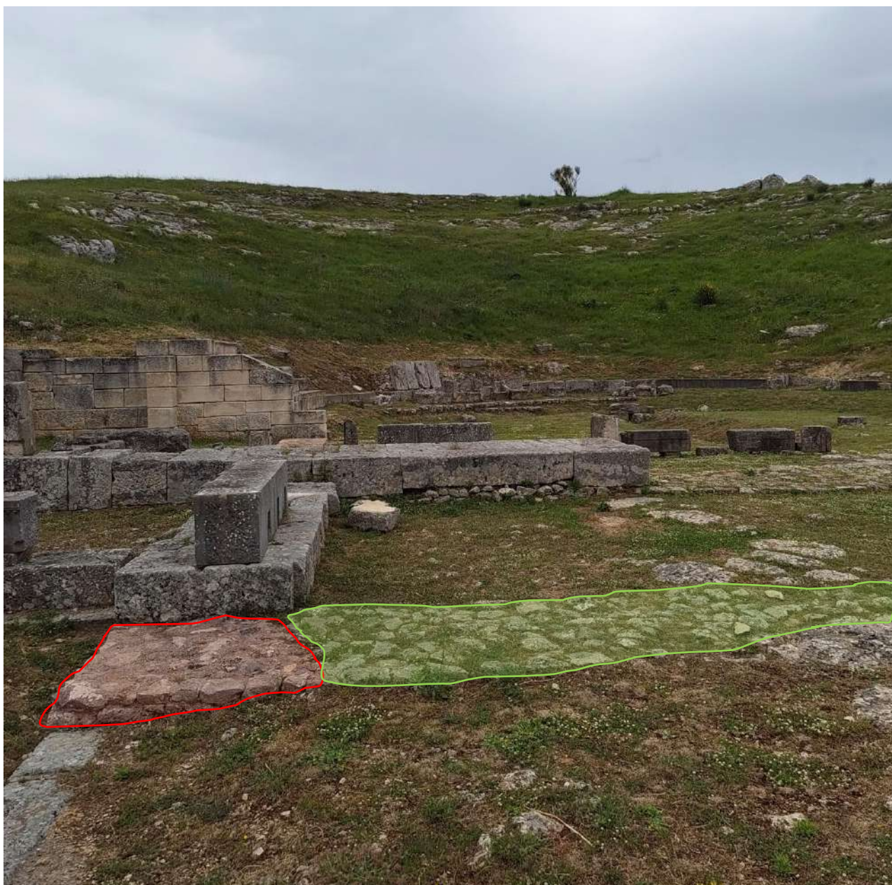
Figure 25 Incomplete cementitious joint repointing, facilitating vegetation growth and loss of archaeological legibility.
