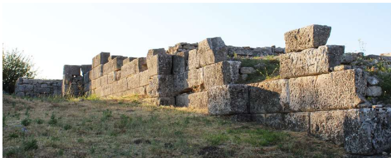
Figure 28 Diateichisma as supporting wall of Stoa
