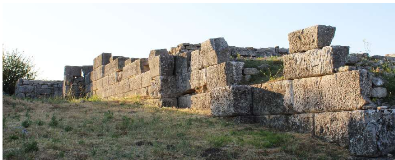
Figure 24 Diateichisma as supporting wall of Stoa
