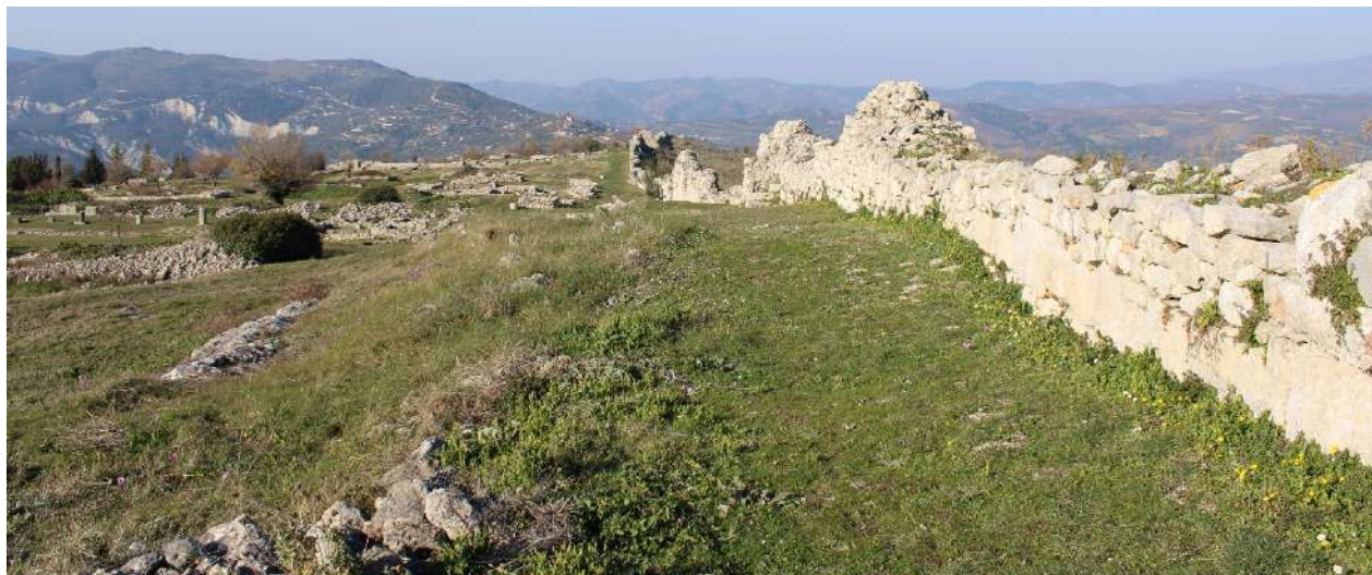
Figure 91 The wall between towers V and X
