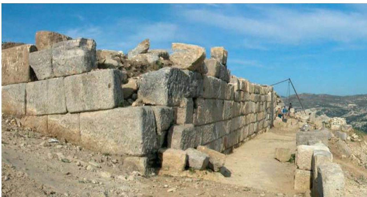
Figure 5 The Gate nr. 1. During the restoration works. Photo by N. Ceka
