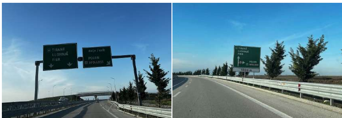
Figura 12 Horizontal and vertical Road traffic signage
