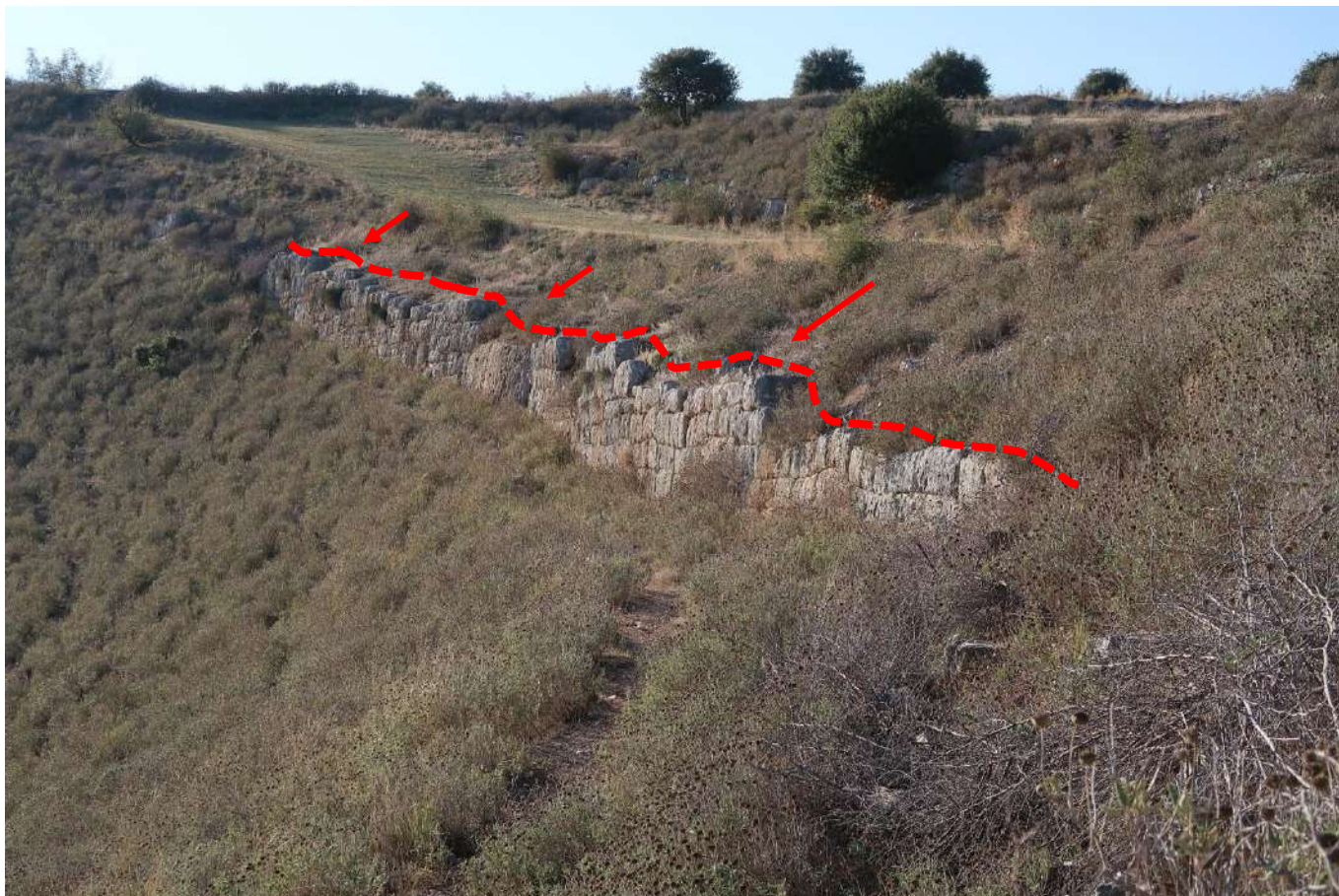
Figure 14 Ancient walls of Klos largely illegible due to insufficient maintenance and site management; risk of soil pressure and slippage.
