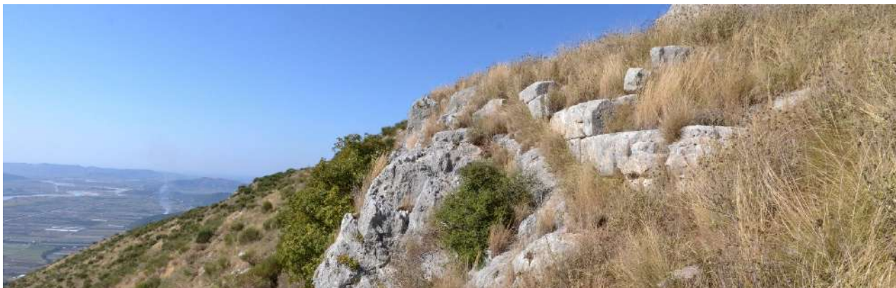
Figure 11 The southern wall
