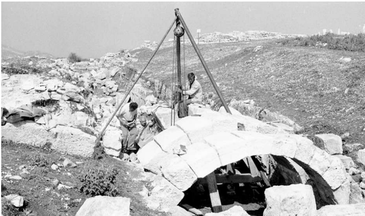
Figure 38 Restoration of the cistern's arches. L. Papajani 1987
