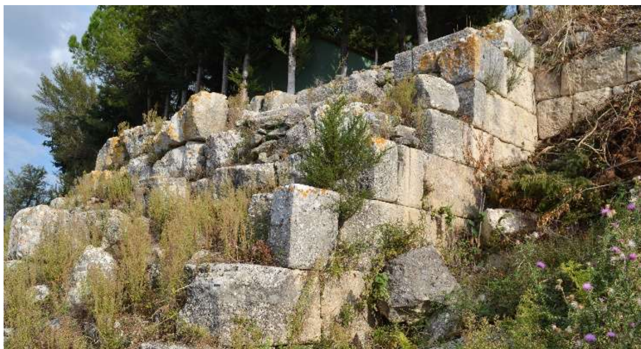
Figure 16 The tower under the Bektashian sanctuary
